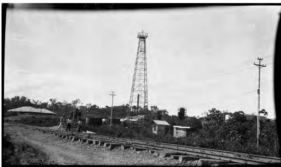
[Infraestructura petrolera de la Tropical Oil Company], Barrancabermeja, c. 1924.
